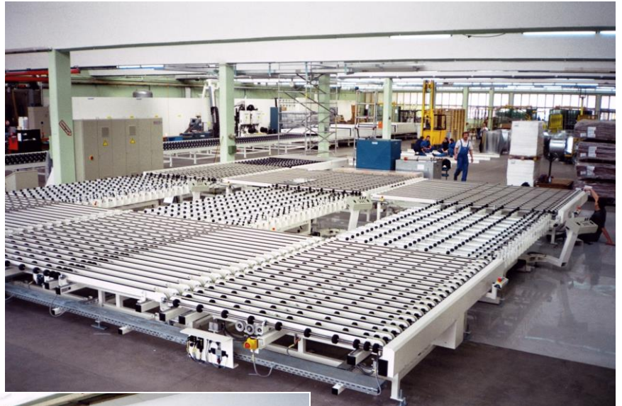
Flachglas-Förderanlage Flat glass-conveying plant
